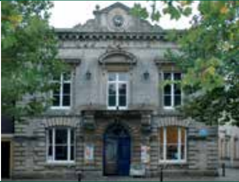
Property of the Town Council; occasionally open.
